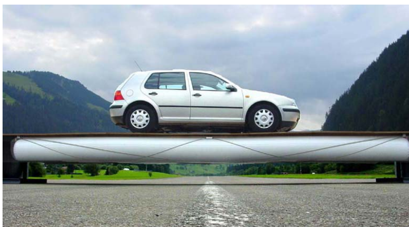
Figure 5. Tensairity demonstration bridge with 8 m span and 3.5 tons maximal load.
